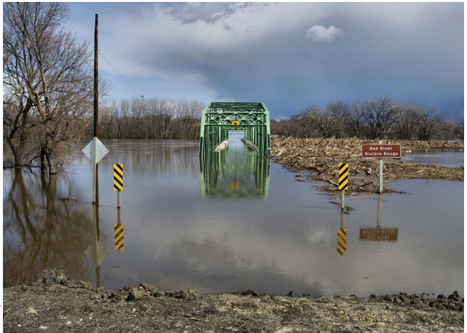
Flooded bridge along the Red River, Manitoba, Spring 2011
